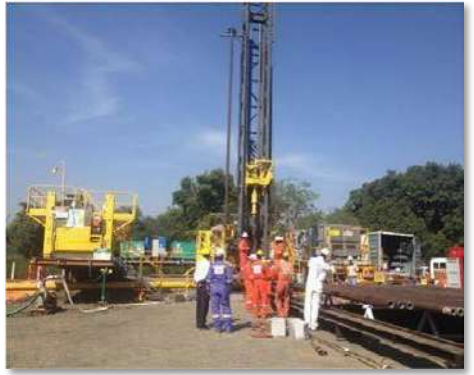
CBM Production Drilling At Sohagpur, MP For Reliance Industries
