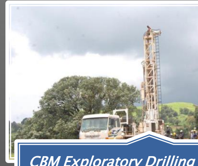
CBM Exploratory Drilling at Satpura, MP for Dart Energy
